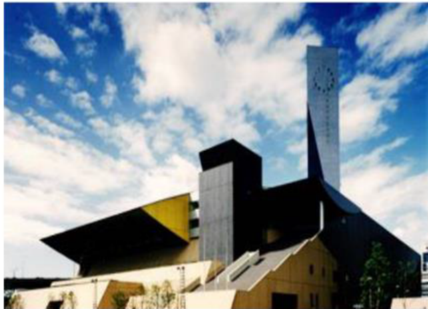
Ariake Incineration Plant
