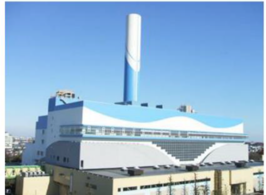
Katsushika Incineration Plant
