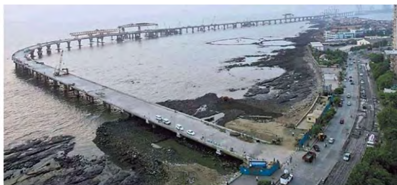
施工中 (RisingCitizen, Sep 6, 2010)
