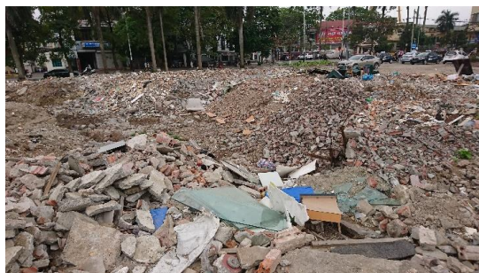
▲Discarded roof tiles and bricks
