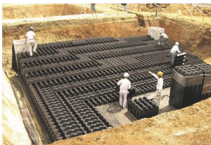
▲ Installation of CROSS-WAVE
