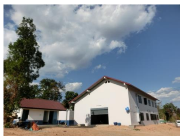
▲Paksan district water purification system building
