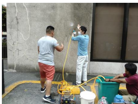
▲ Applying Ever Prolong
