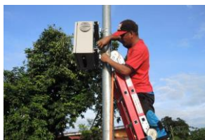
▲Installation of Alarm Unit (City of Iloilo)
