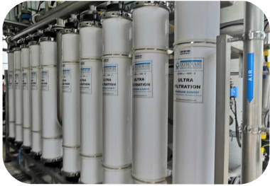
Water Efficiency to reduce average water intake to 2.6 liters in water-stressed areas
