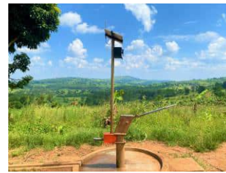
▲ Installation of SUNDA system
