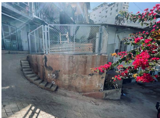
▲ Completion of landslide countermeasure works by well and drilling in Dalat city
