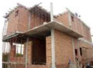
House under construction (Vietnam)
