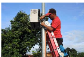
▲Installation of Alarm Unit (City of Iloilo)
