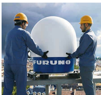
▲Installation by hand
