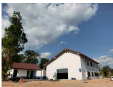
▲ Paksan district water purification system building
