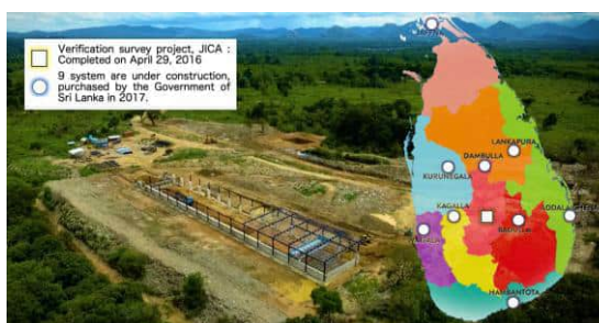
▲ 9 system are under construction
