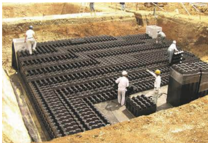
▲ Installation of CROSS-WAVE
