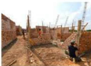
House under construction (Indonesia)
