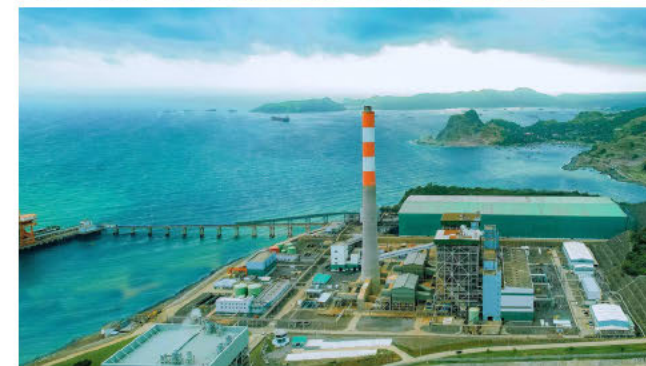
GMEC (GNPower Mariveles Energy Center)
