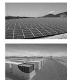
400 MW Solar + Storage
