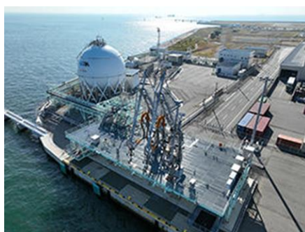
Figure 14 Liquefied Hydrogen Terminal (Hy touch Kobe) (Source: HySTRA)
