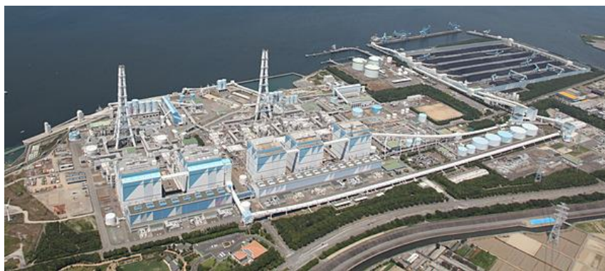
Figure 5 JERA Hekinan Thermal Power Plant (Source: JERA)
