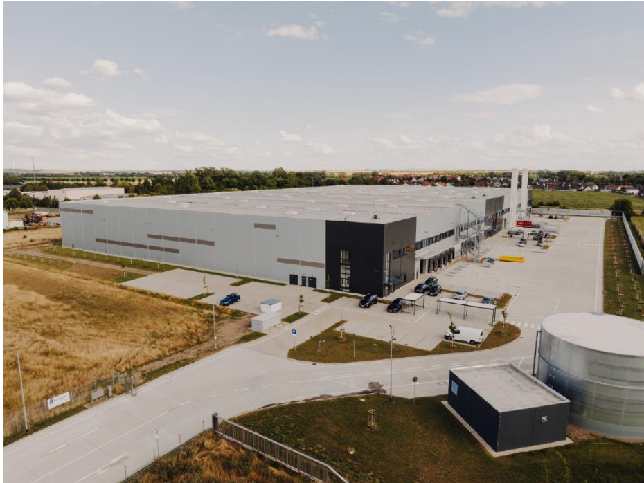
Li-Cycle's first European lithium-ion battery recycling facility, which is located in Magdeburg, Germany, has commenced operations. The Germany Spoke is the largest in the company's portfolio and one of the largest facilities of its kind in Europe.
