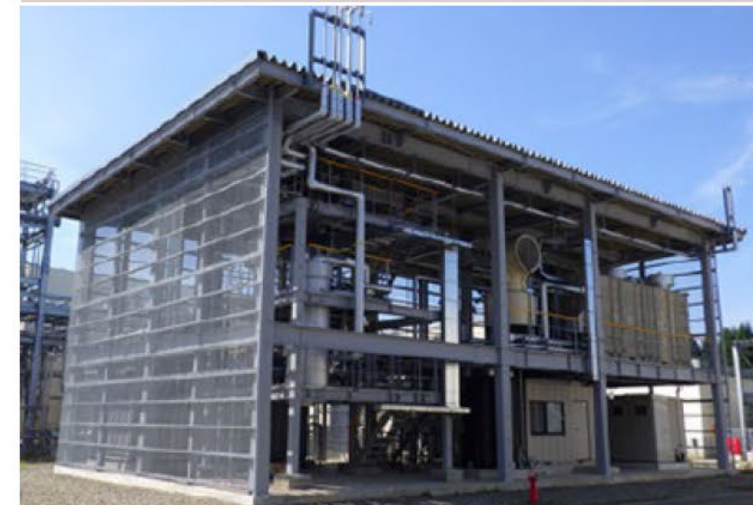
An 8Nm 3 /h class methanation test device created at INPEX Nagaoka Mine
