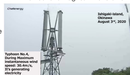
▲ Generated power at 30.4 m/s peak wind speed
