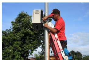
▲Installation of Alarm Unit (City of Iloilo)
