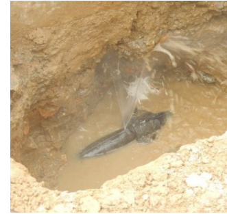
▲Identified water leakage point
