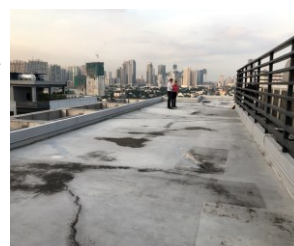
▲ Cracks on a building roof (Philippines)
