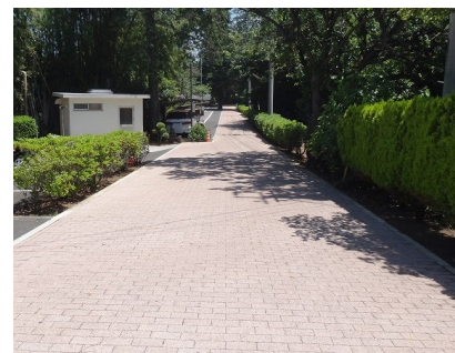
▲ Road paved with waste roof tiles and brick blocks
