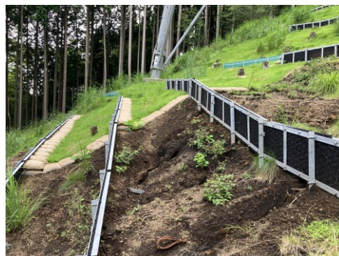
▲ Comparison of SARD method mounted area and non-mounted area
