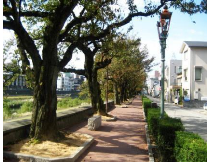
▲ Road paved with waste roof tiles and bricks
