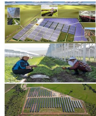
▲ 3 : Chile First Solar Power Plant Power sales started in June 2021
