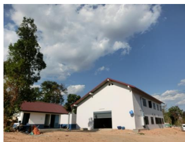
▲ Paksan district water purification system building
