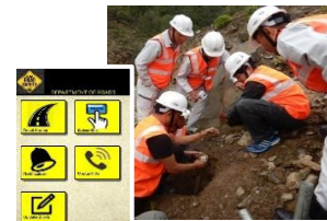
▲ Installation of monitoring sensors for ex-ante traffic control as components of a smartphone-based road information system
