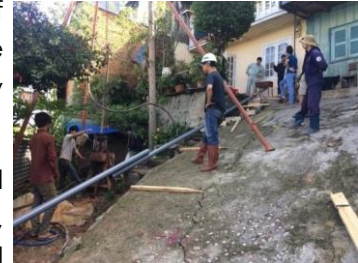
▲Emergency Survey and Installation of Monitoring Post for Prevention of Landslides
