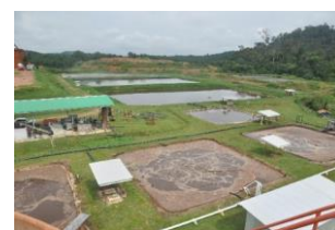
▲Wastewater treatment plant in palm oil factory in Malaysia
