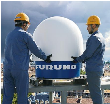
▲Installation by hand
