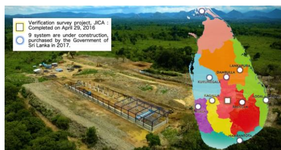
▲ 9 system are under construction
