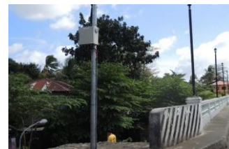
▲Installed Alarm Unit (City of Iloilo)
