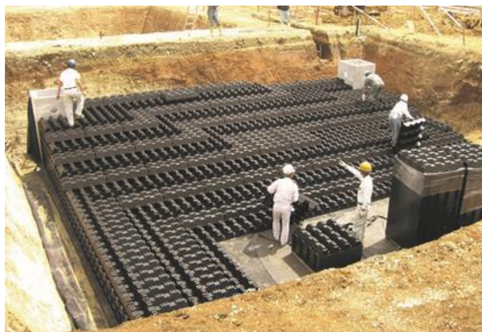
▲ Installation of CROSS-WAVE
