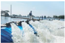
▲ Drainage works by the Japan Disaster Relief Team
