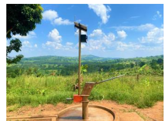
▲ Installation of SUNDA system
