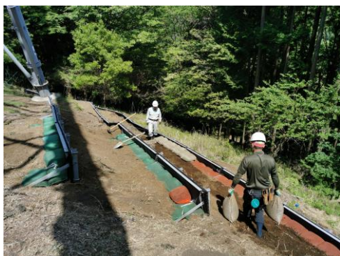
▲SARD method mounting work (green: volcanic ash, red: coal ash)
