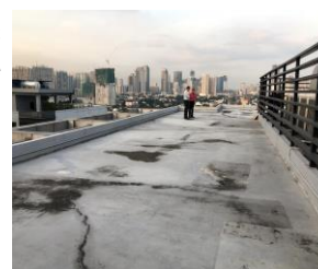
▲ Cracks on a building roof (Philippines)
