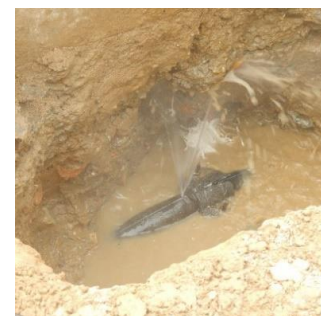
▲Identified water leakage point
