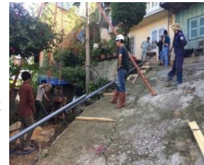
▲Emergency Survey and Installation of Monitoring Post for Prevention of Landslides
