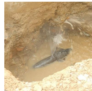
▲ Identified water leakage point
