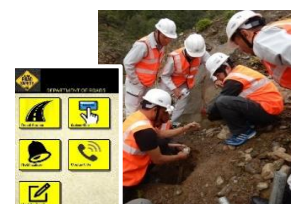
▲ Installation of monitoring sensors for ex-ante traffic control as components of a smartphone-based road information system
