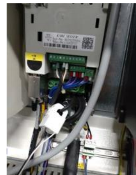
CT sensor ( electrical current sensor )
