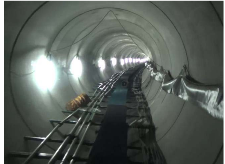
3.5m width 1.3 km length tunnel × 2 under 15m
