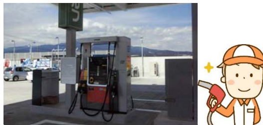
Vapor recovery facility
