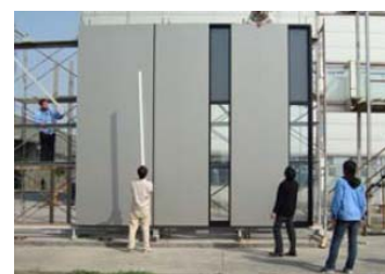
Inspection of aluminum curtain wall
