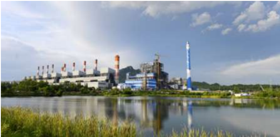
Mae Moh Coal-Fired Power Plant, which is the subject of the biomass co-firing study.
