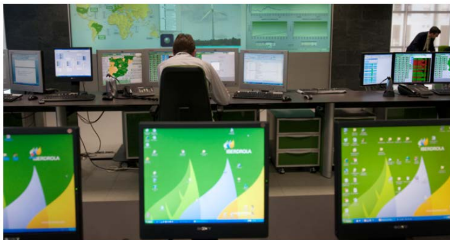
Renewable Energy Operations Centre (CORE), Toledo (Spain).
