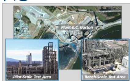
Figure 1. Photographs of Post-Combustion Carbon Capture Test Facilities
