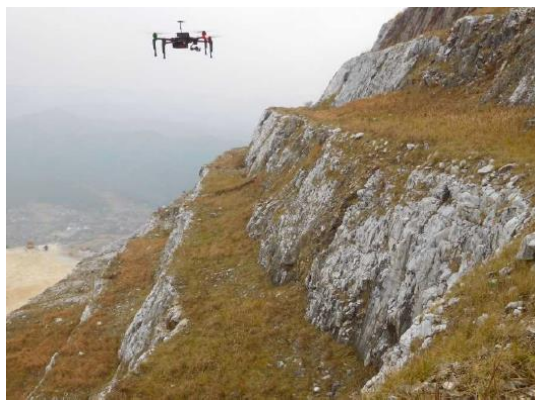
残壁の浮石点検
